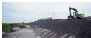
Noise barriers in the Netherlands made of slag Source: CEWEP 2011
